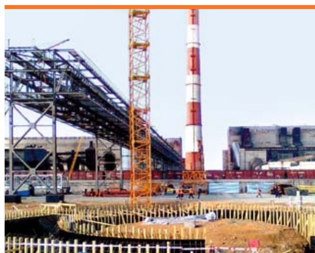
Construction and installation works. Reftinskaya GRES
