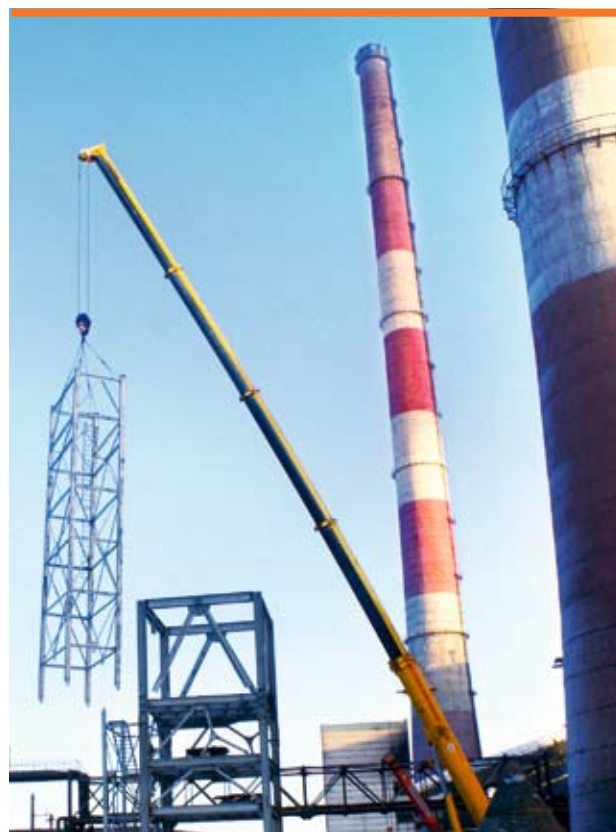
Construction and installation works. Troitskaya GRES
