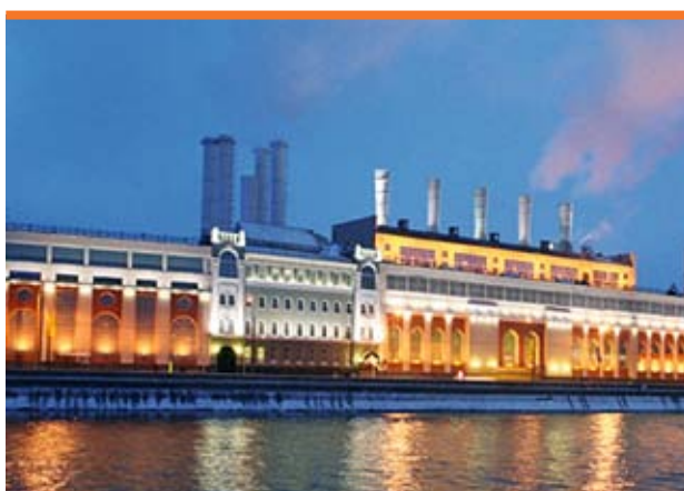
Hydro Power Plant GES-1, Mosenergo.
